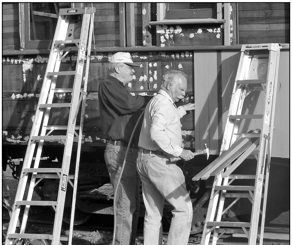
Roger Sherman (left) and Bob Tully install siding on the Rico. – Photo © Denny Haefele.
