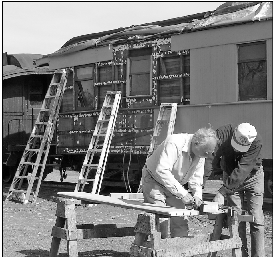
Bob Tully (left) and Roger Sherman work on siding for the Rico. – Photo © Denny Haefele.
